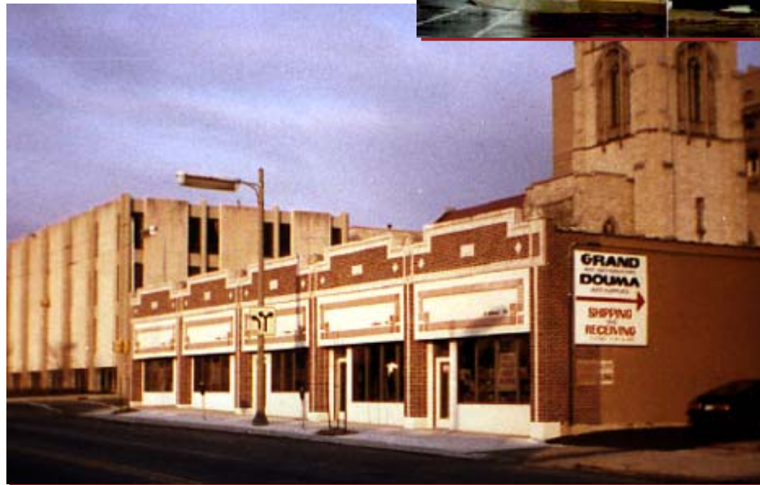
NEW PHOTO MAIN ENTRANCE AFTER RENOVATION
