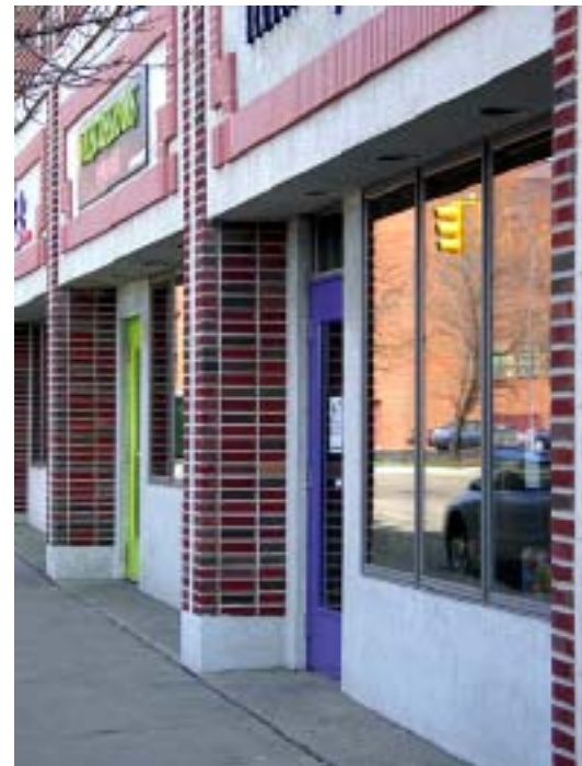
View looking at the new store front recess.
