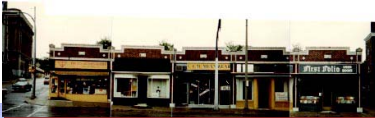
EXISTING PHOTO BEFORE RENOVATION
