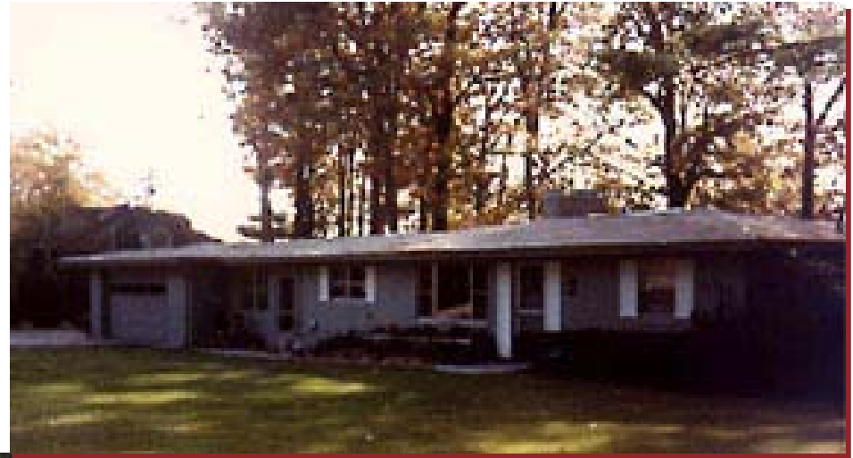
EXISTING PHOTO MAIN ENTRANCE BEFORE RENOVATION
