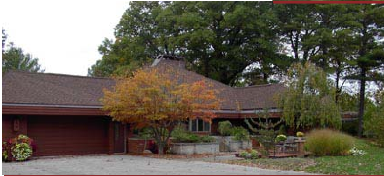
NEW PHOTO MAIN ENTRANCE AFTER RENOVATION
