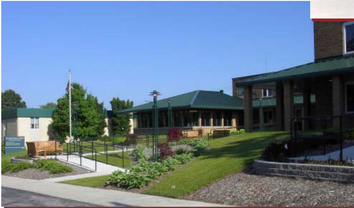
NEW PHOTO MAIN ENTRANCE AFTER RENOVATION
