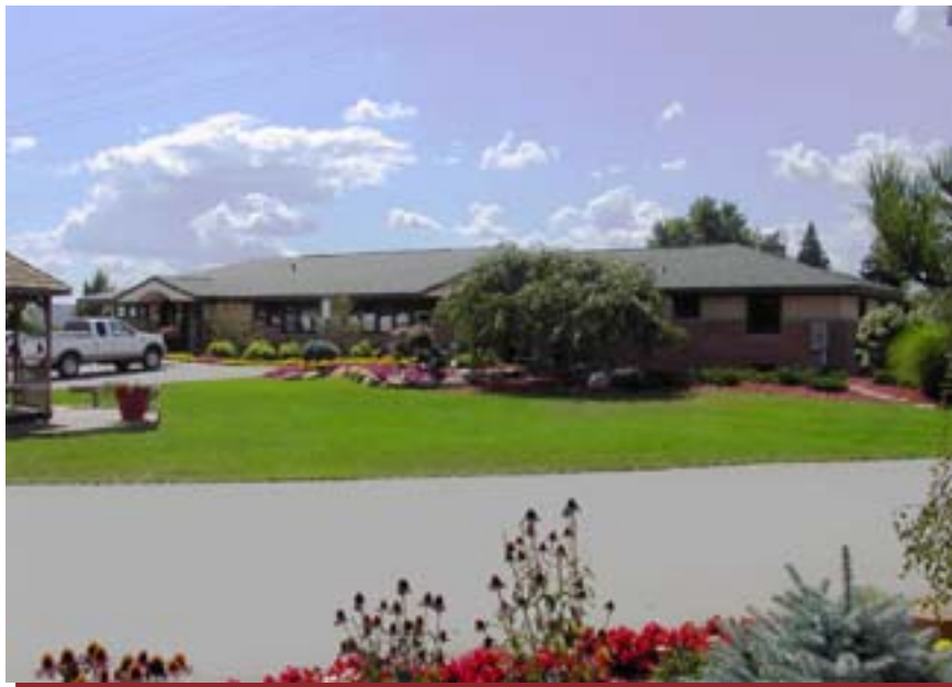
VIEW LOOKING AT THE NEW OFFICE ENTRANCE FROM THE EAST SIDE LOOKING WEST.
