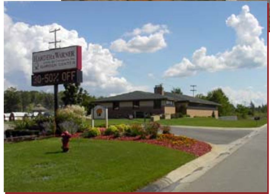
VIEW LOOKING SOUTH AT THE WEST WALL OF THE NEW OFFICE BUILDING
