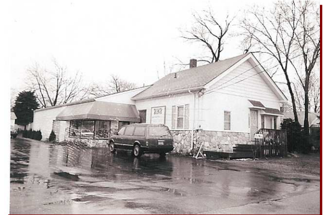
EXISTING PHOTO MAIN ENTRANCE BEFORE
