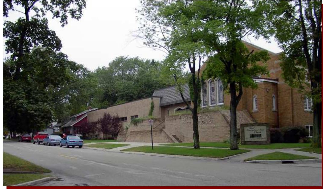
View of the MAIN ENTRANCE after the renovation
